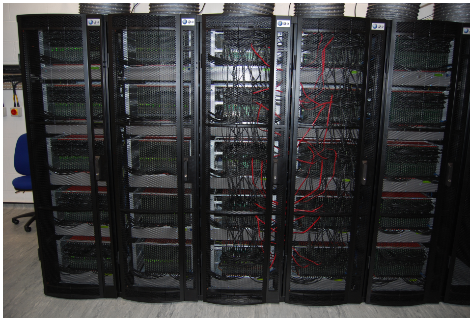
Figure 3: SpiNNaker system used for the NCP
