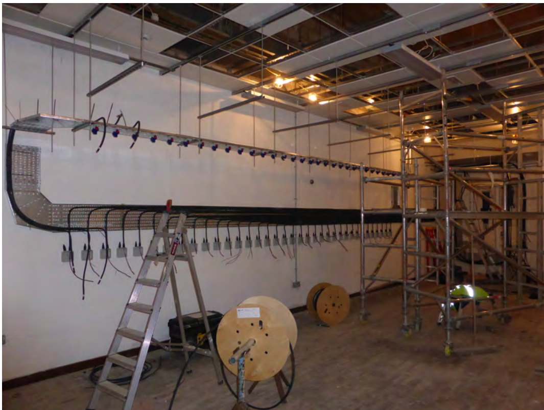
Figure 14: The room currently being prepared for the full scale NM-MC1 machine
